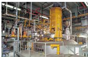
● Interior of the MX Plant
